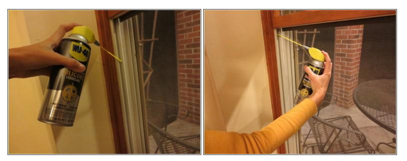
• Apply a thin coating of the silicone spray onto the windows' channels.
