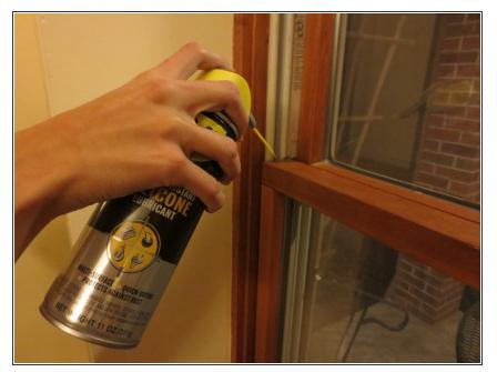
• Apply the silicone spray where the window and channel connect if the window is stuck.
