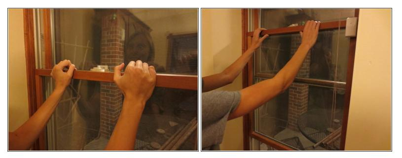
• Slide the window up and down along the channel until the silicone spray is evenly distributed.
