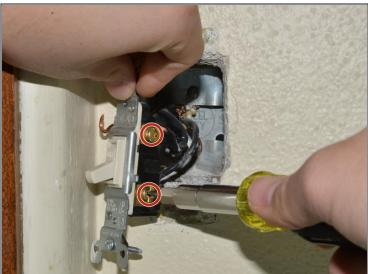
Unhook the wires from the screws.
