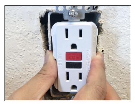
Push the outlet and wires back into the wall.
