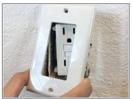
Using #2 flat-head screwdriver, remove the outlet cover by unscrewing the top and bottom screw.
