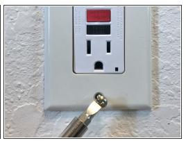
Install the outlet cover by tighten the top and bottom screws.
