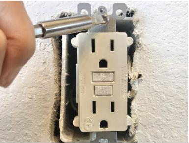
Using #2 flat-head screwdriver, unscrew the top and bottom screws holding the outlet onto the wall.
