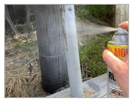
• Paint the upper and lower assemblies for prevention of future rust and corrosion.
