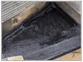
• There was a lot of oil/dust sludge beneath the oil cooler, requiring a rather dirty cleanup.
