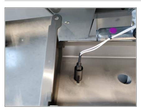
Connect the white cables to the ignitor.
