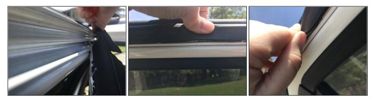
• Press the weatherstripping firmly into its seated position.
