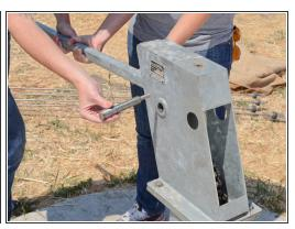
While supporting the pump handle, remove the axle.
