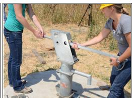
Slide the pump handle out of the pump head.
