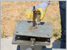
Remove the spacer from around the pump rod.
