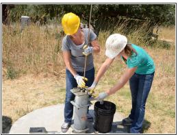
Loosen the rod clamp and repeat the procedure for the next section of pump rod.
