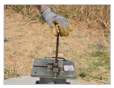
Screw the jam nut back onto the top of the pump rod.
