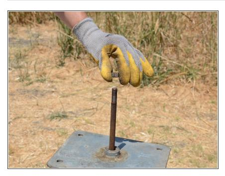
Remove the jam nut from the top of the pump rod.
