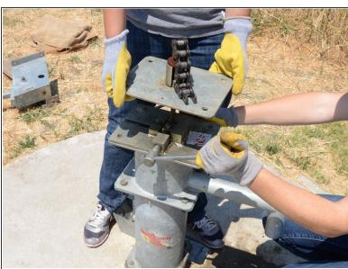
Tighten the rod clamp against the pump rod.
