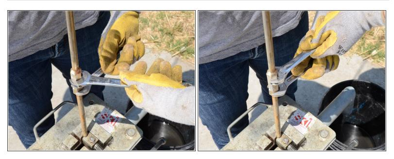
Use two wrenches to loosen the joint between the top section of pump rod and the rest of the pump rod.
