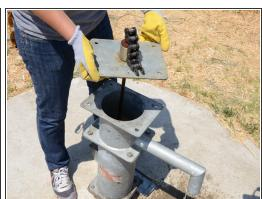
Lift the head flange up about one foot above the tank.
