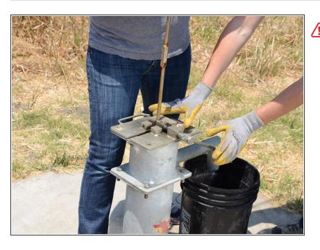
Be sure the rod clamp is tightened against the pump rod.
