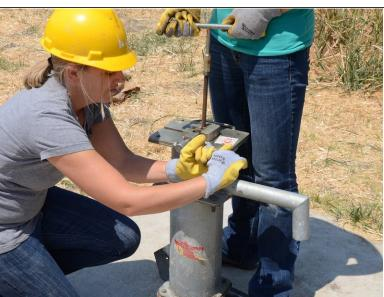
• Have one team member lightly pull up on the T-handle, while another loosens the rod clamp. This will prevent damage to the pump.
