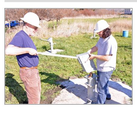
Lift the pump head off of the water tank and place in a sanitary place, preferably above ground, to prevent contamination. To reassemble your device, follow these instructions in reverse order.
