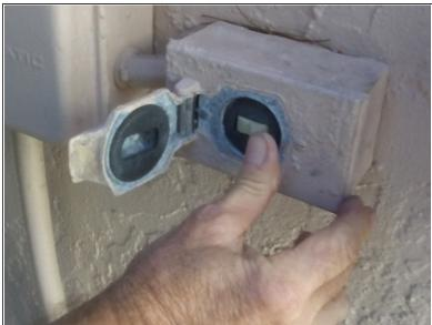
Make sure the pool pump switch is off.
