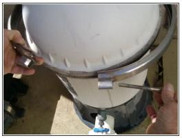
• Unscrew the metal ring bracket that is on the filter housing in order to remove the top half of the filter housing (lid). Turn the handle in a counter-clock wise motion until it is completely loose and the screw can be removed.
