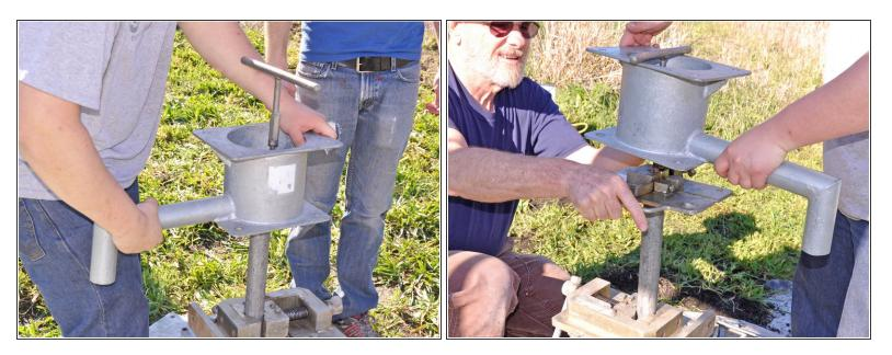
• Turn the water tank counterclockwise until it comes free from the pipe.
