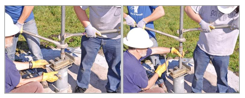
• When you reach the pipe coupling, open the clamp more to allow it to pass through. Lift the riser main approximately one foot above the clamp and re-secure the pipe.
